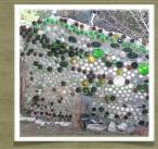
Foundation Preparation: Trench 12-18 inches deep and 6 to 8 feet long with supports on either side- preferably railroad ties. Fill trench with rocks or cement blocks and concrete Let foundation set up and harden before beginning first course of bottles. (a day or so, as it depends on the humidity in your area) Organize bottles-larger ones interspersed with smaller:
